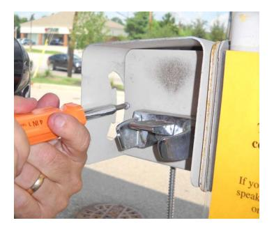
2. Disconnect the RJ12 plug from the RJ12 coupling, and then bundle and secure excess wires with the zip tie provided.
