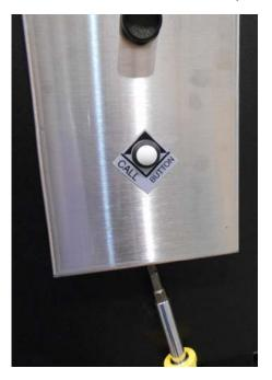
Unplug the existing panel microphone and call button wires from the harness in the frame.
