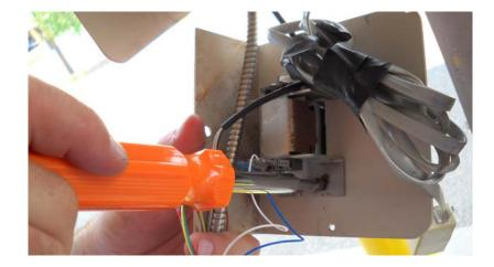
4. Remove nuts to disassemble the handset cable block from the back plate.
