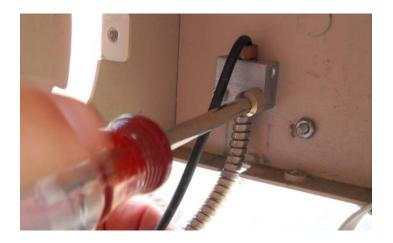
5. Assemble the retrofit cradle assembly to the faceplate. Feed the wire through the cut out in the faceplate and secure the cradle using nylon locking nuts provided.
