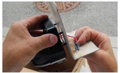
6. Install the new handset assembly by attaching the new handset cable block to the studs in the back plate using the nuts removed in step 4.
