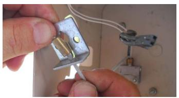
8. Install the handset pigtail to the existing harness by connecting the RJ12 plug into the RJ12 coupling.
