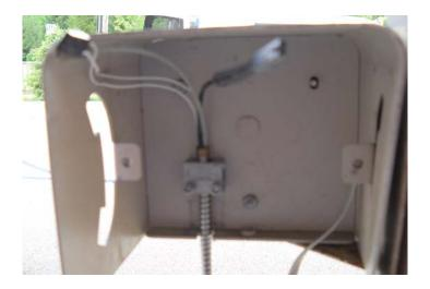
7. Insert the safety lanyard cable into the backside of the cable restraint and pull down to seat. Install the cable restraint onto the top right stud of the back plate using a nylon locking nut.
