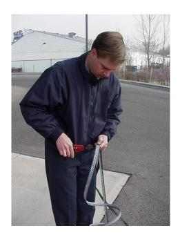
Use the old tape to measure and cut the new tape.
