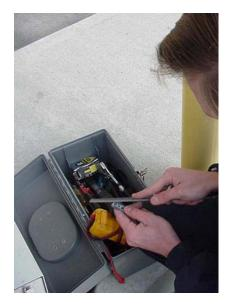
Bevel and round the ends of the tape with a file. See page 10 for the correct configuration of the tape ends.
