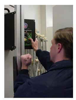
Go inside to the vertical unit. Insert a small screwdriver into a hole in the tape. Press and hold the brake release button on the brake control board. Pull down on the screwdriver feeding the tape around the sprocket. Continue to due this until the carrier is resting on the stabilizers outside. (Be careful that the carrier has not caught on the speaker wires).
